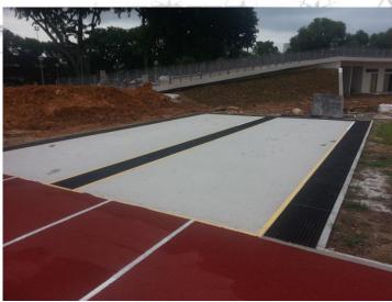
40420: Aluminium sand traps prevent sportsmen from spreading sand into the running track, when they are leaving sand pits. Sand can cause damage to synthetic surfaces. Aluminium sand trap is made from special aluminium profiles. The trap also includes aluminium grates and honey rubber mat. Aluminium sand trap can be installed singly or as a double row. It measures a length of 1 m and a width of 50 cm.
